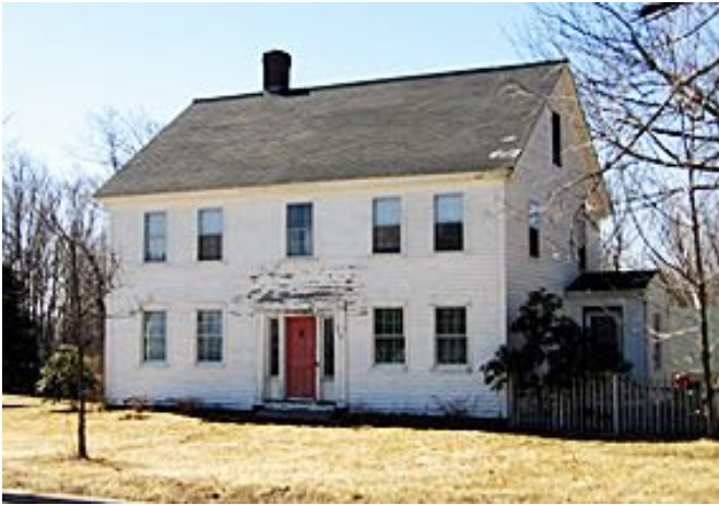
(Photo 1) - The Corner of Hubbardston Rd. & Boylston Ave
