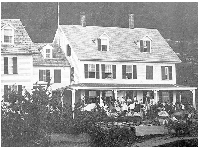
Photo 5) - Mountain House at 261 Mountain Rd
