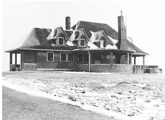
(Photo 22) – Henry C. Delano Built in 1902 - 58 Mountain Rd. Site of First Meeting House
