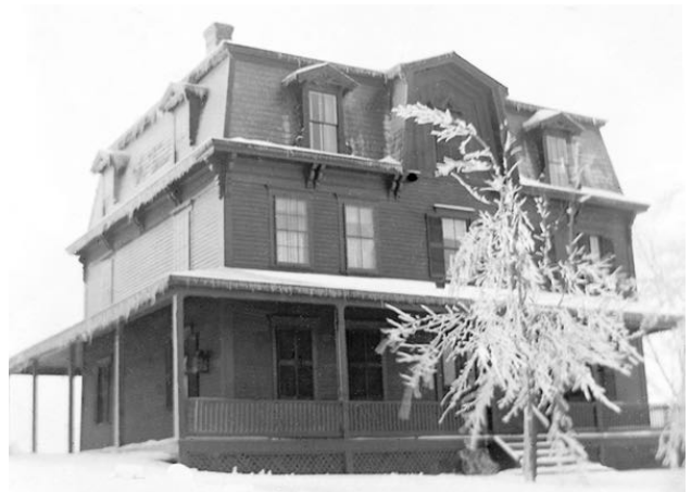
(Photo 2) - Wachusett House Tavern After Move & Expansion - 7 Boylston Ave
