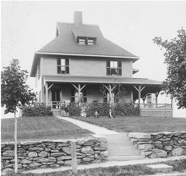
(Photo 19) – A. G. Bullock Built in 1870's - 10 Worcester Rd.
