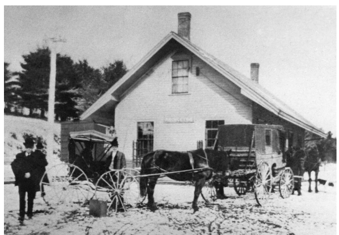
(Photo 12) – Princeton Depot 1875 - 283 Hubbardston Rd.
