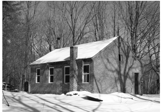
Schoolhouse #6 on Schoolhouse Rd off Ball Hill Rd. demolished and rebuilt as a private home.
